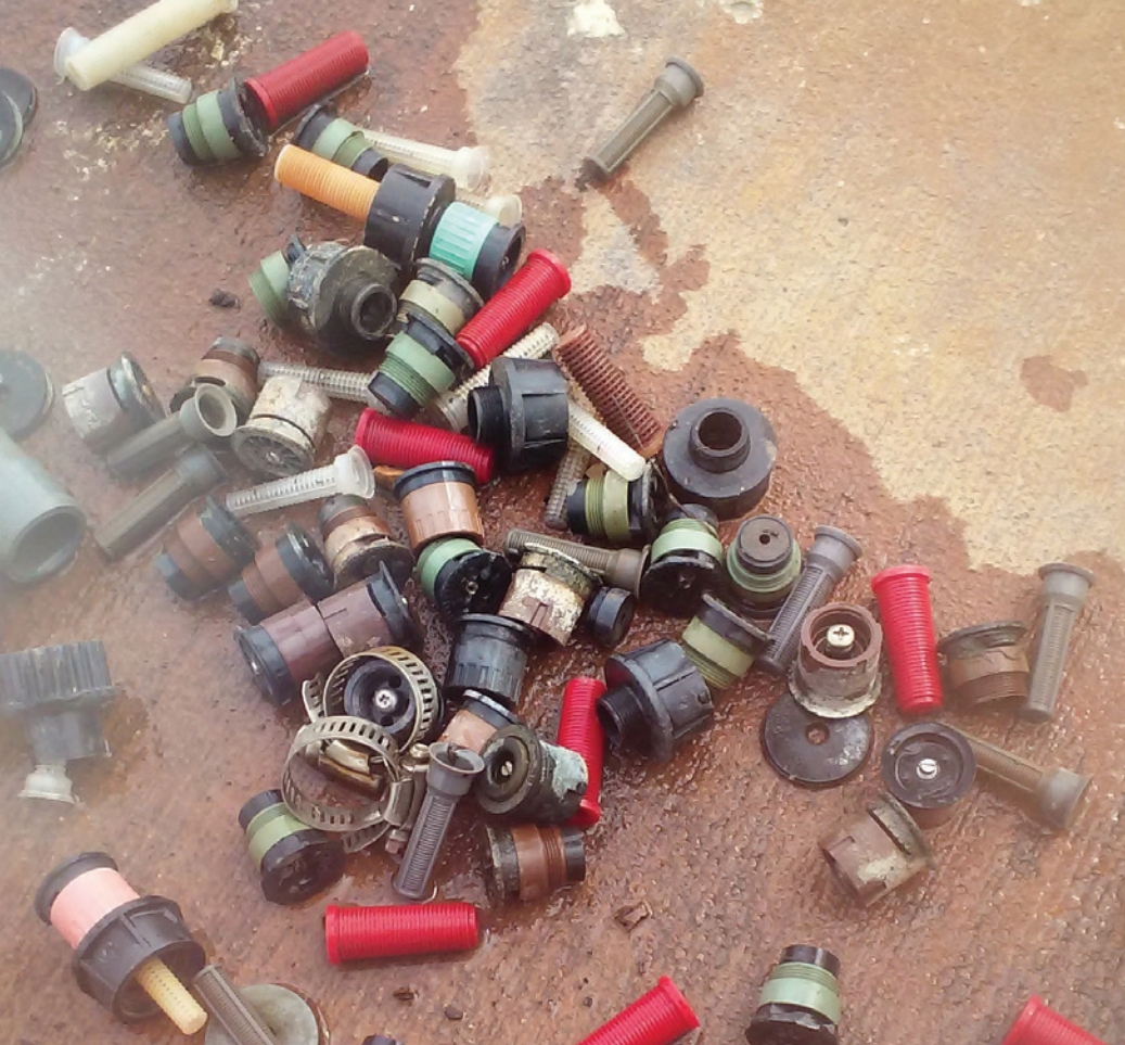
Figure 3 – Different stages of iron residue (orange) on irrigation heads and filters. Residue from calcium carbonate (white) can also be seen. Note the orange color of the sidewalk, a result of constant irrigation with high iron water.
