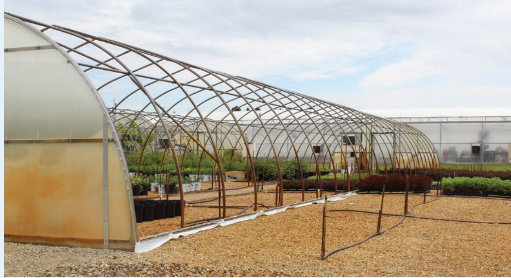
Figure 4 – Iron residue at the MSU research nursery. The rock groundcover was white limestone that has now turned bright orange after years of irrigating with high iron water. Also note the residue built up on the end wall and hoop ribs.
